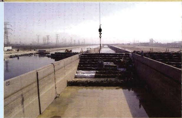
INSTALLATION OF SANDBAGS @ SUPPLY CANAL
